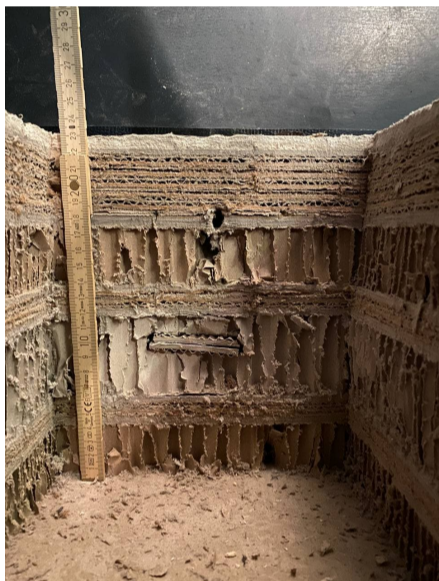
Floor component opening (left), position of the measurement sensors (right). TUDa 2023.
